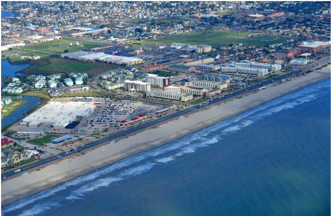
Figure 3.22 Pre- and Post-construction (Top and Bottom) Photos in Project's East-Central Area
