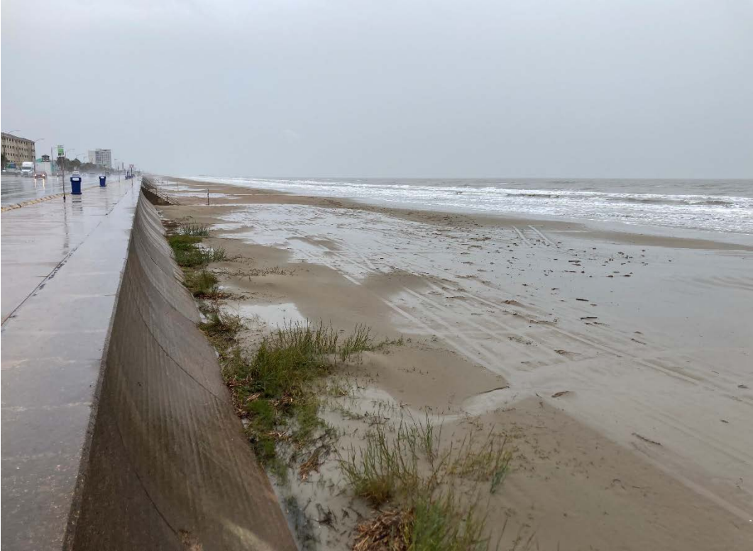
Figure 3.32 Existing Conditions on November 21, 2022 at West End of Fill Taper
