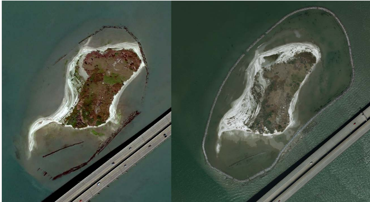
Figure 4.10 Causeway Rookery Island Pre- and Post-construction (source: GLO)
