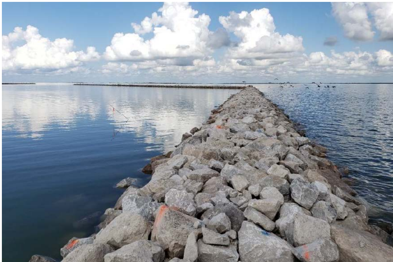
Figure 4.3 Typical Post-construction Breakwater Conditions, December 2021 (HDR, 2022)
