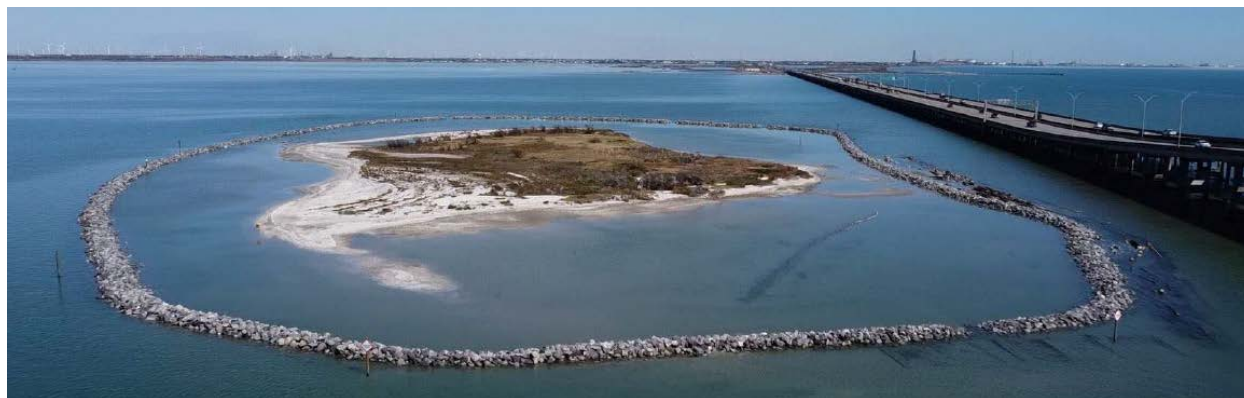
Figure 4.12 Northeastward View of Completed Project in 2022 (source: GLO)
