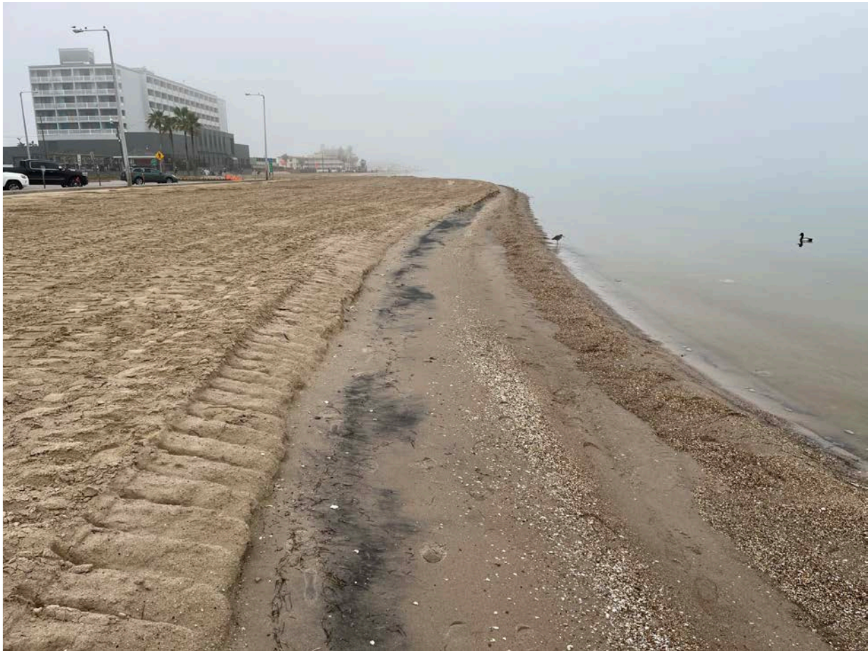
Figure 3.13 North Beach Post-Construction Conditions (Looking North) (December 2022; provided by GLO)
