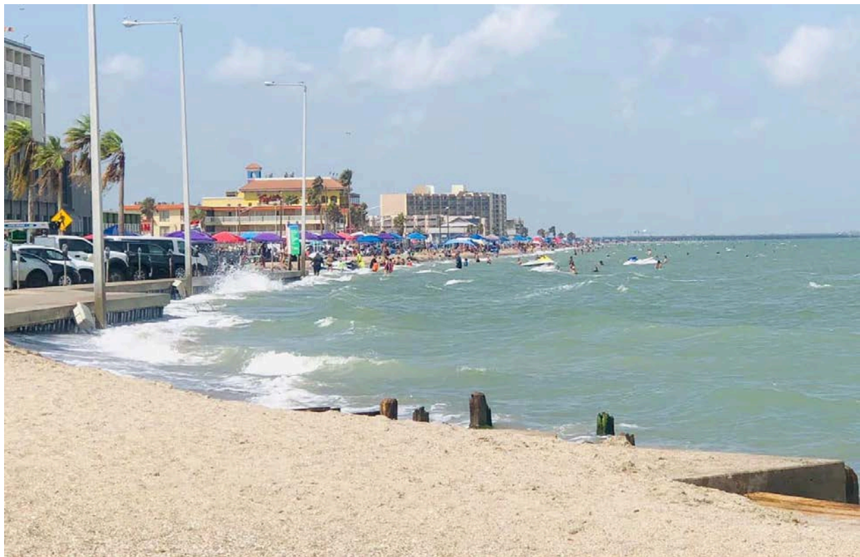
Figure 3.12 North Beach Pre-Construction Conditions (Looking North) (August 2022; provided by GLO)
