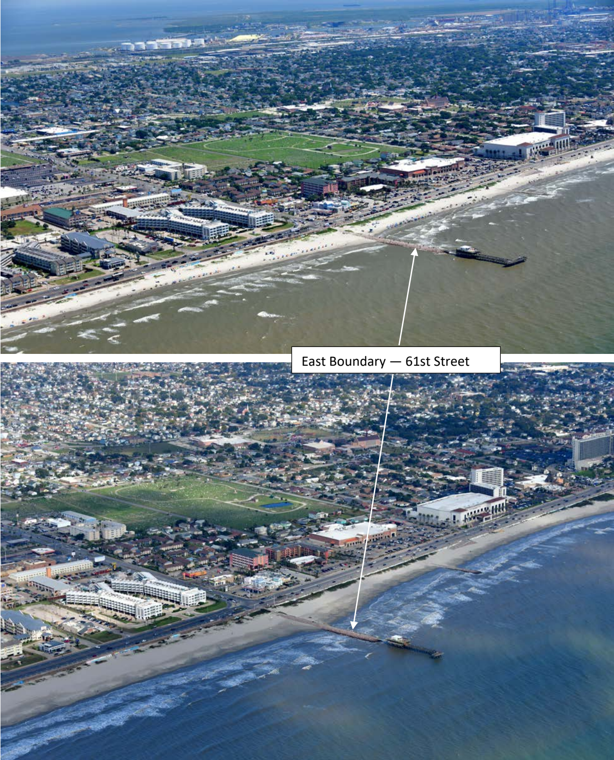
Figure 3.21 Pre- and Post-construction (Top and Bottom) Photos at Project's East End
