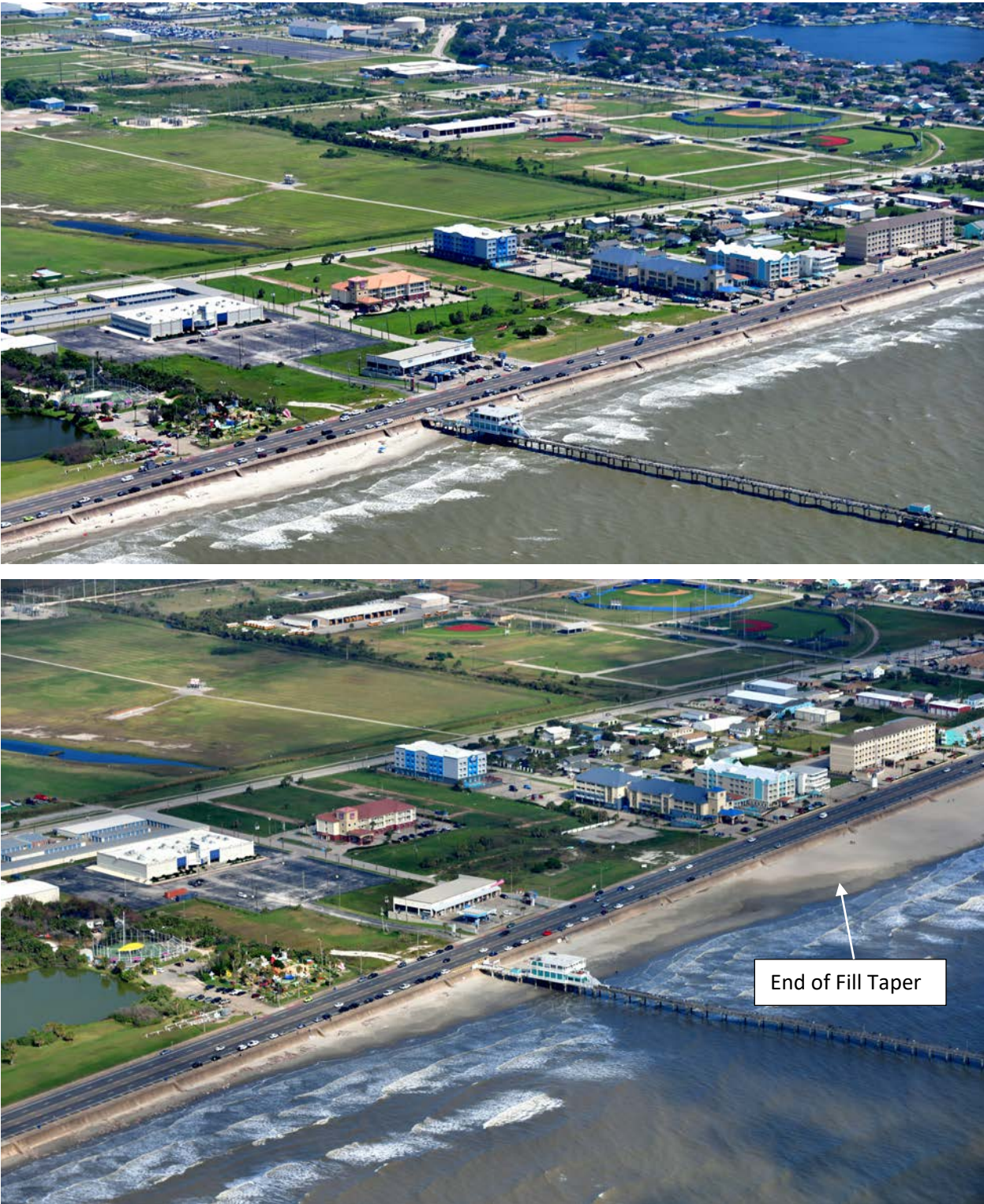
Figure 3.25 Pre- and Post-construction (Top and Bottom) Photos at Project's West End
