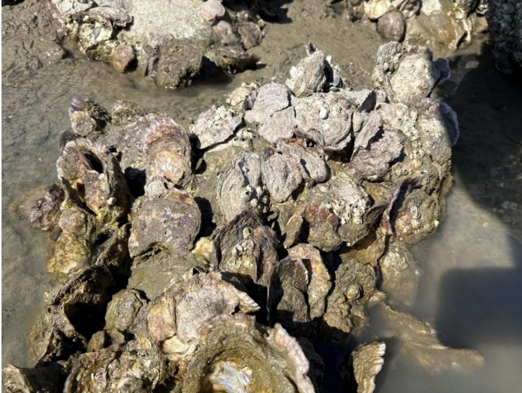
Figure 14. Oysters and barnacles on Butterowe Bayou breakwater.
