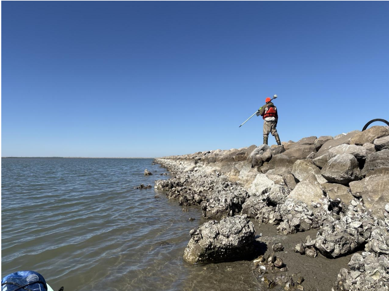
Figure 6. RTK GPS measurement of the Oak Bayou breakwater crest elevation. Photo facing northeast.
