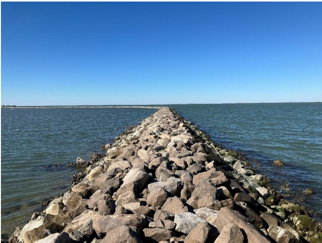
Figure 4. Typical ground digital photograph of the crest of the Oak Bayou Breakwater (facing west).
