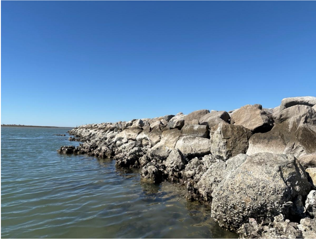
Figure 3. Typical ground digital photograph of the base of the Oak Bayou Breakwater (facing west).
