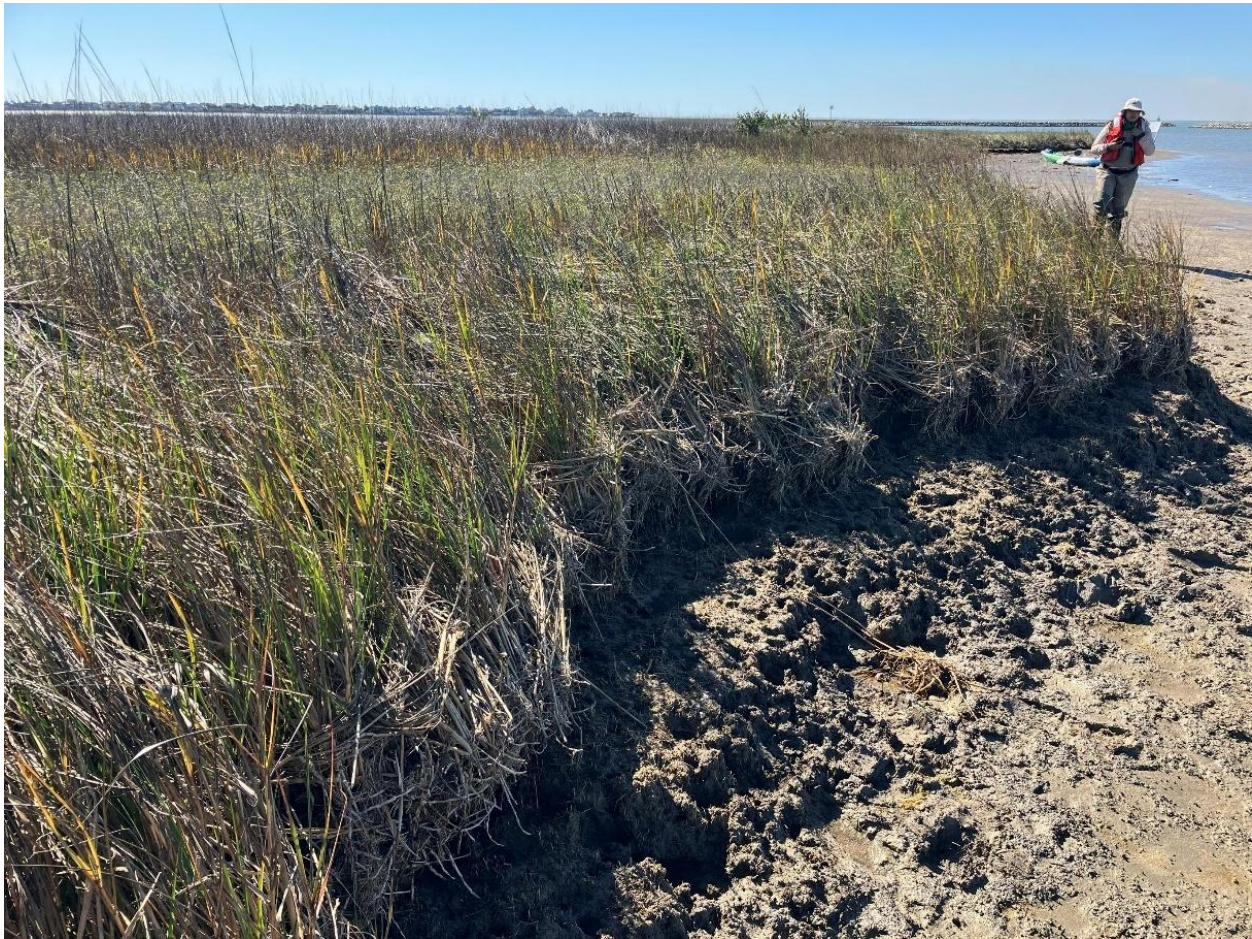
Figure 17. Vertical scarp along marsh shoreline at Area A.
