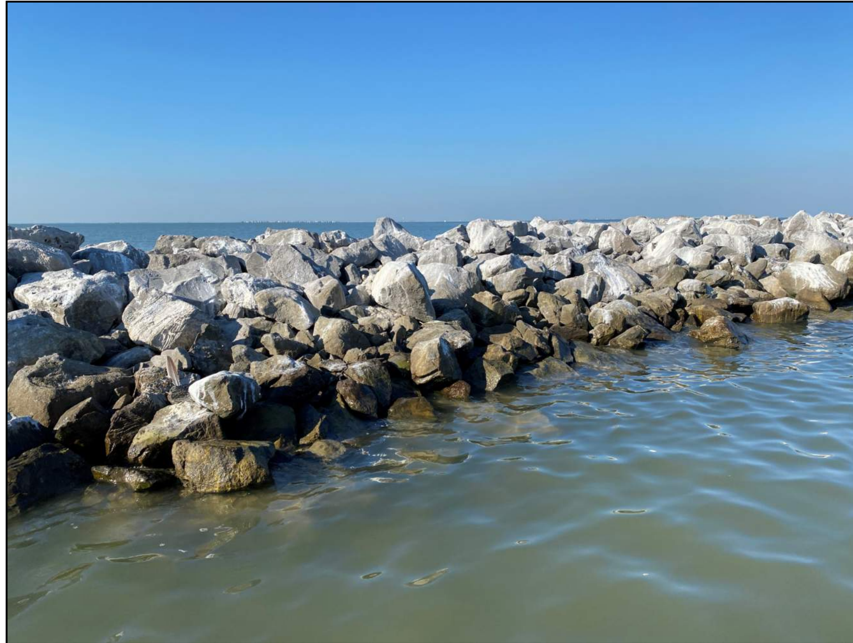
Figure A81. Area A: Breakwater2
