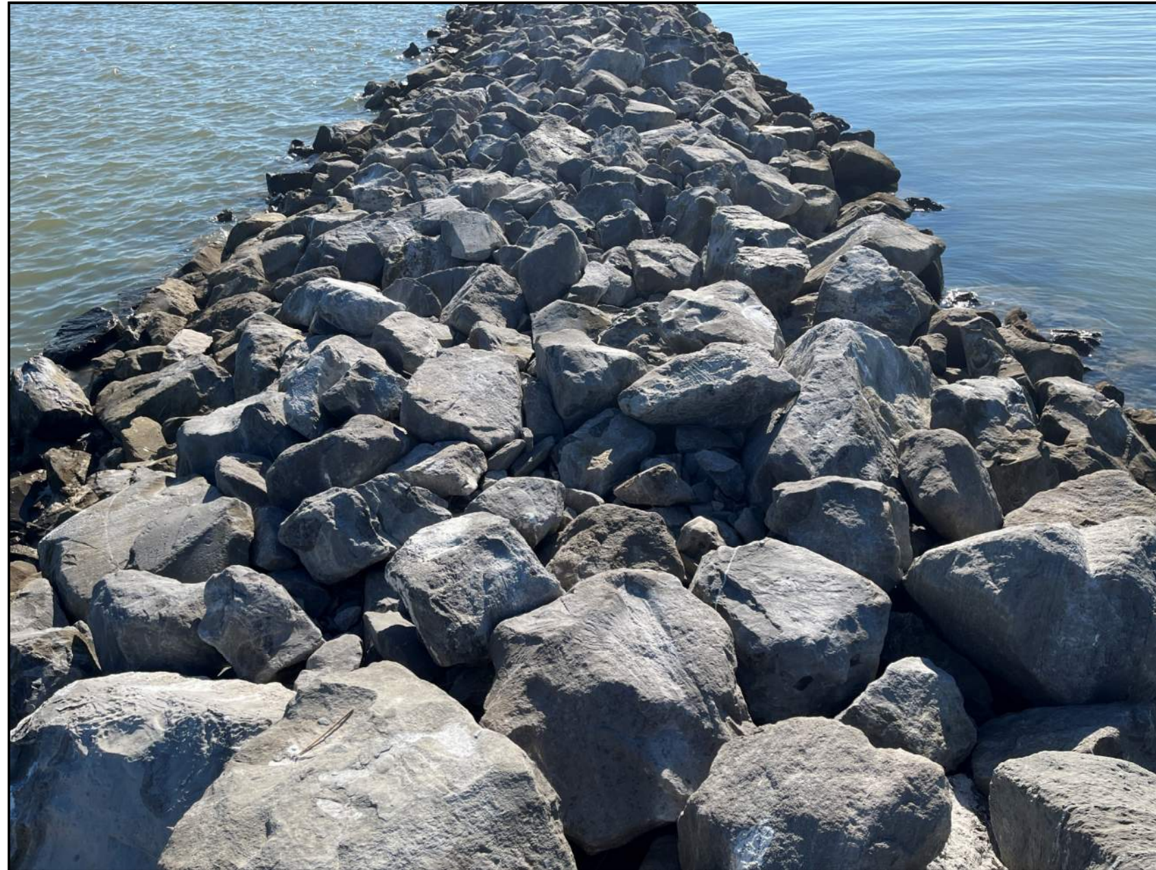
Figure A80. Area A: Breakwater1
