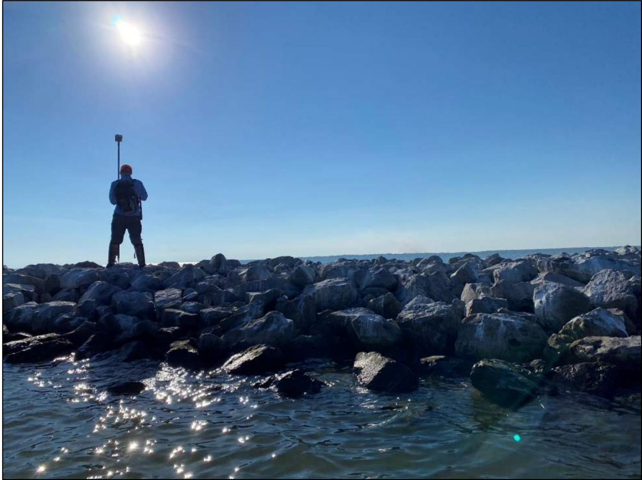
Figure 9. RTK GPS measurement of the Carancahua Cove breakwater crest elevation. Photo facing northeast.
