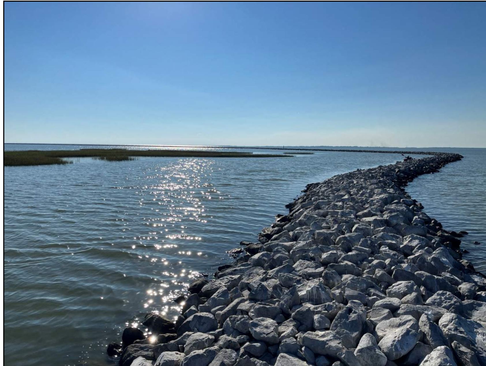
Figure A82. Area A: Breakwater3
