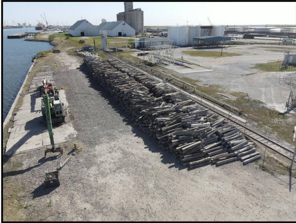
Drone image of stacked railroad ties, material handler at left
