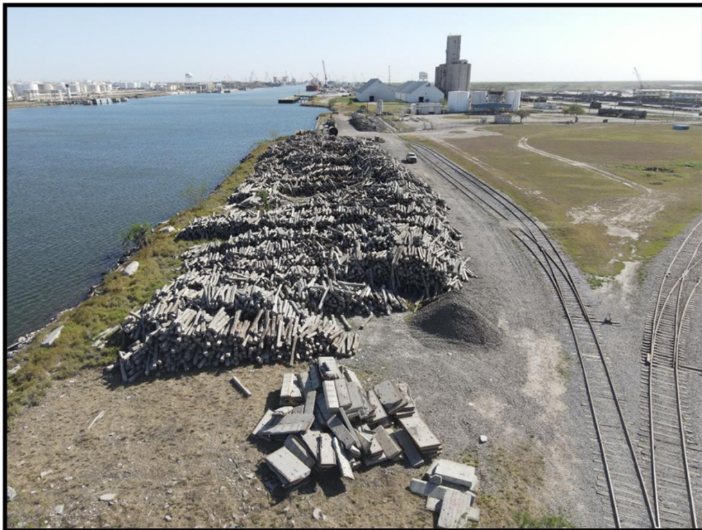
Drone image of stacked railroad ties and concrete blocks
