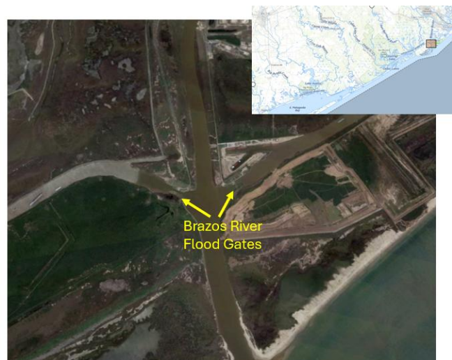
Figure 1-8: Brazos River Flood Gates at the intersection with GIWW.
