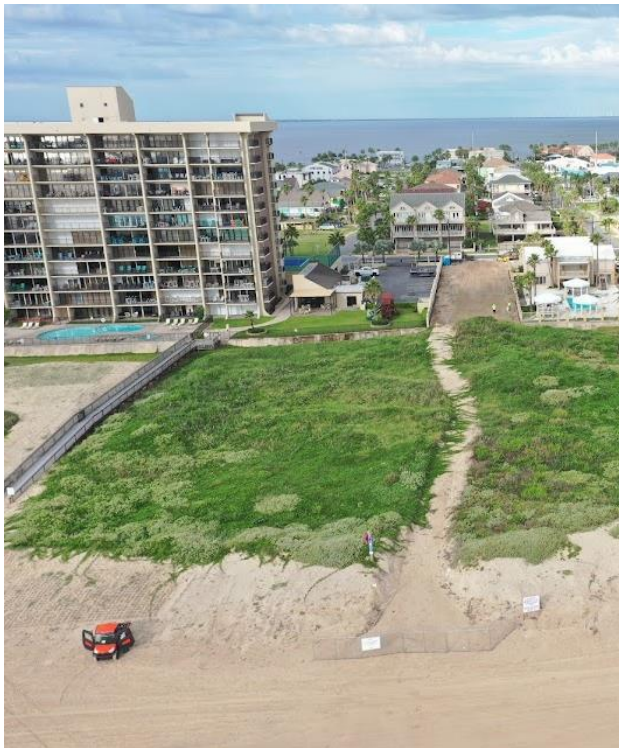
Figure 4. Sloping and sand placement
