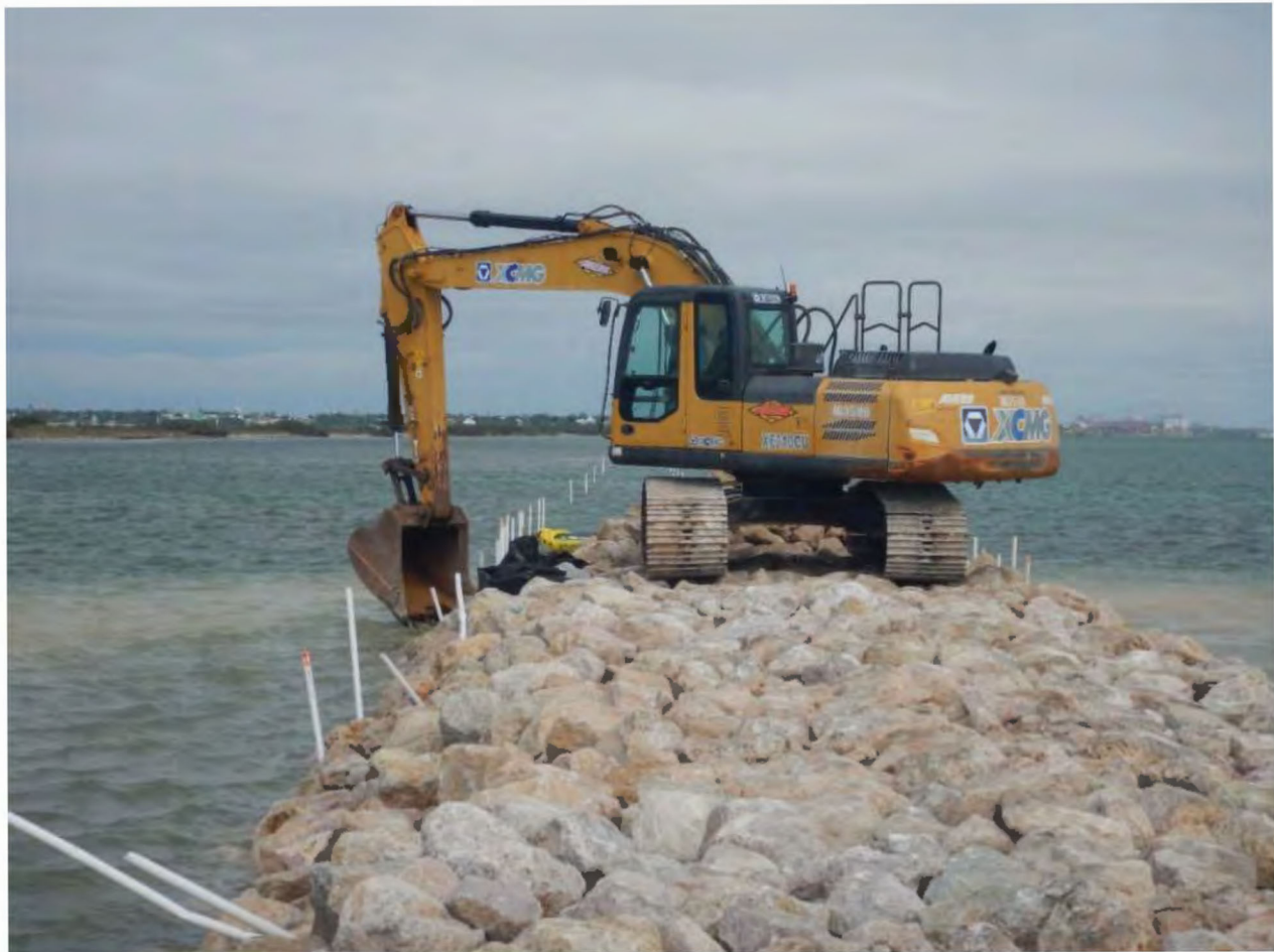
Figure 15. End-on breakwater construction
