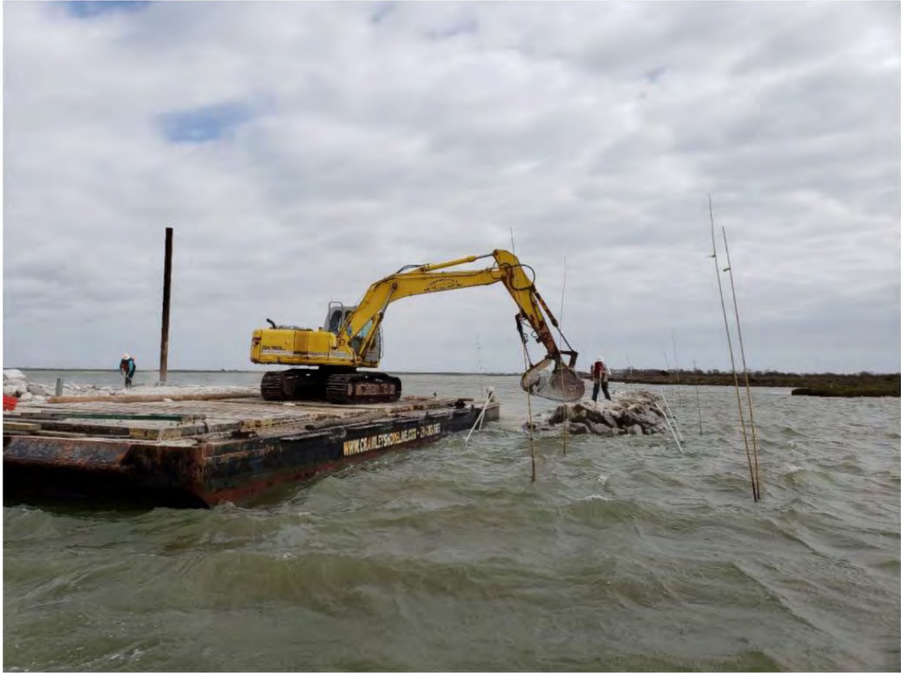
Figure 14. Breakwater construction by light loaded barges
