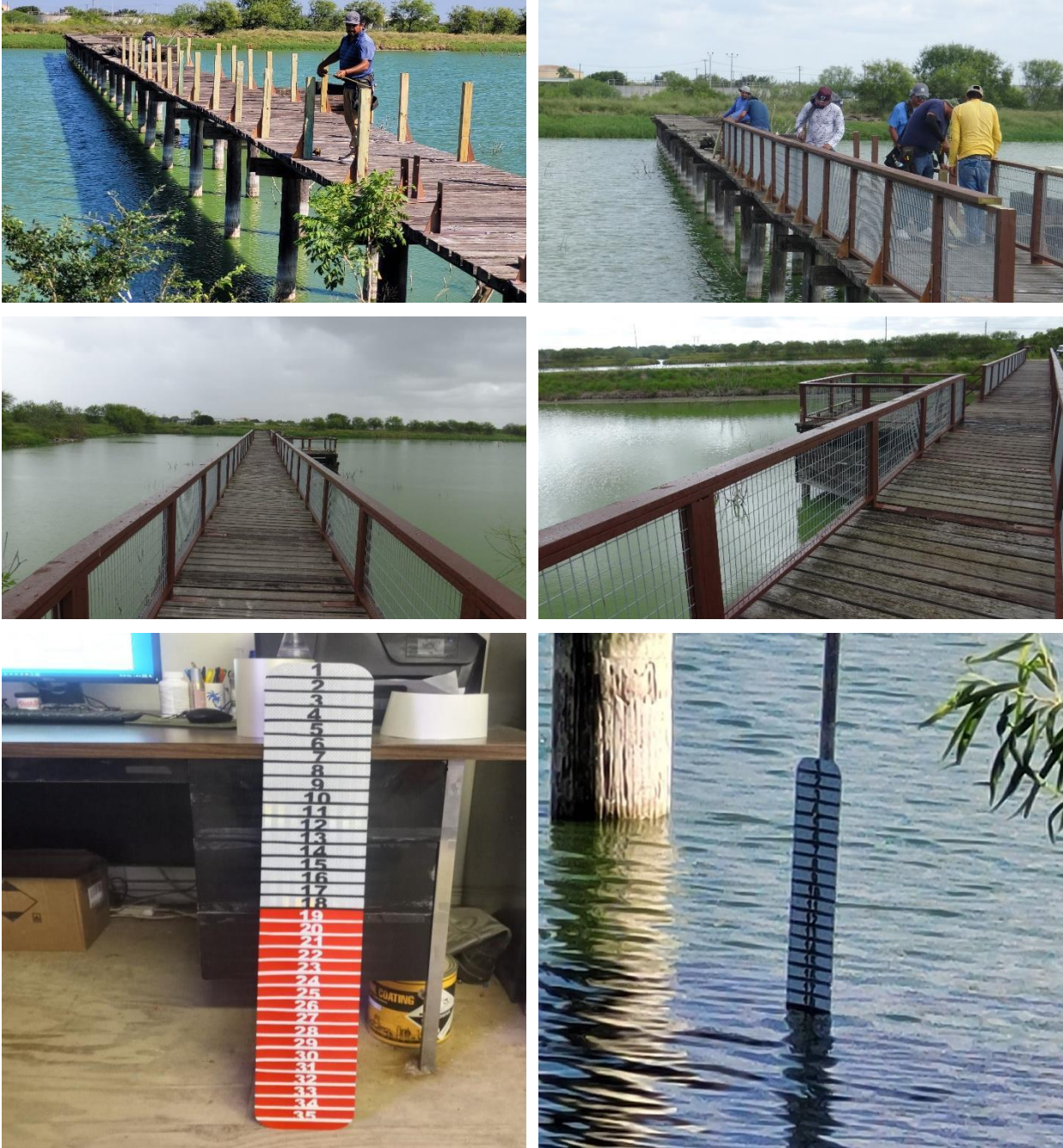
Photos of the pier renovation and water level gage installed in large wetland cells
